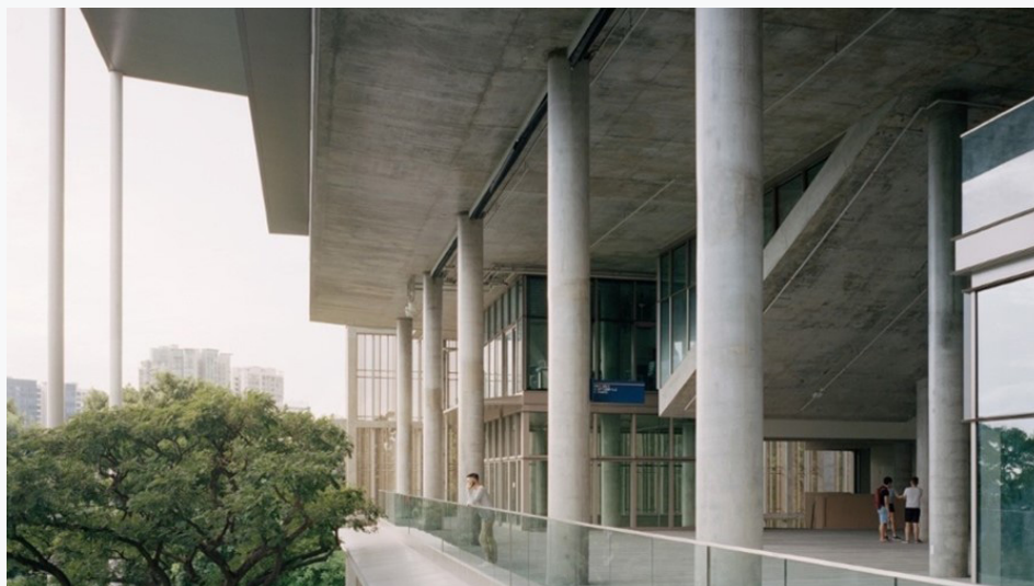
Opening in 2019, the SDE 4 building at the National University of Singapore is the first new-build net-zero energy building in the nation. It features the use of efficient HVAC systems, solar photovoltaics, and architectural designs suited to a tropical environment. (Source: Kevin Hsu)
